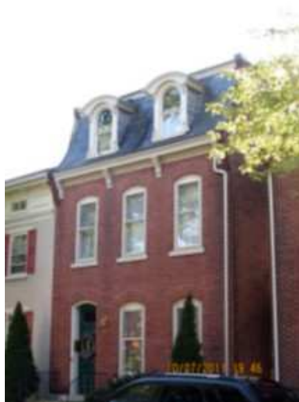
Mansard roof at 217 N. 3 rd St. Photo by Tom Greaves
