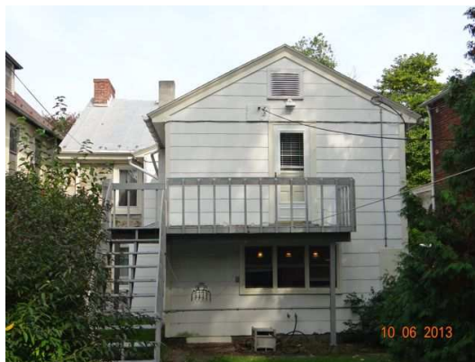
37 S. Water St. from the rear yard, showing the conjoined frame building.
