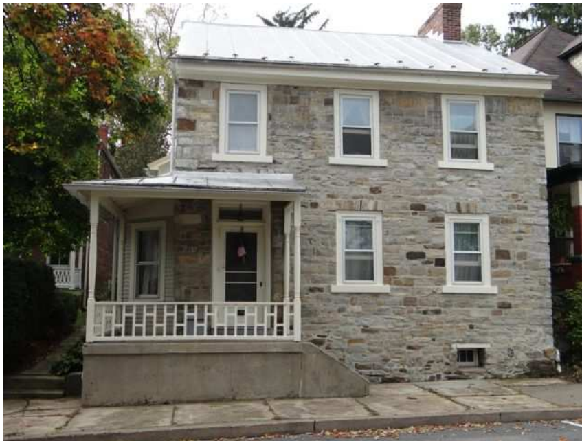
The William Williams House, 37 S. Water St., Lewisburg 1786
