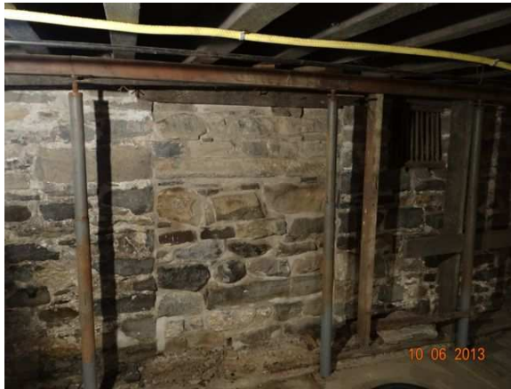
Walled in basement doorway in the wall facing Water Street
