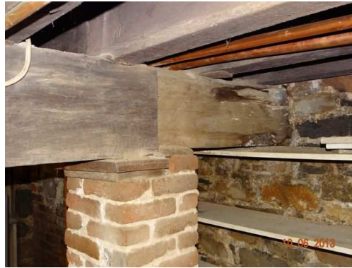
Main basement support beam with replaced end and newer support column
