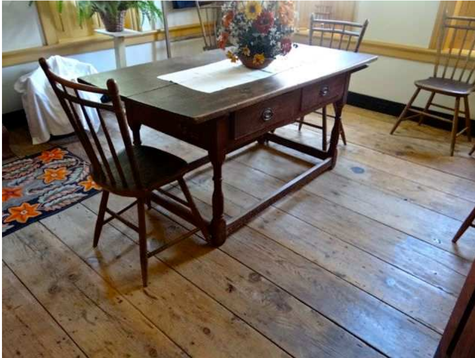
Example of original, unfinished floors
