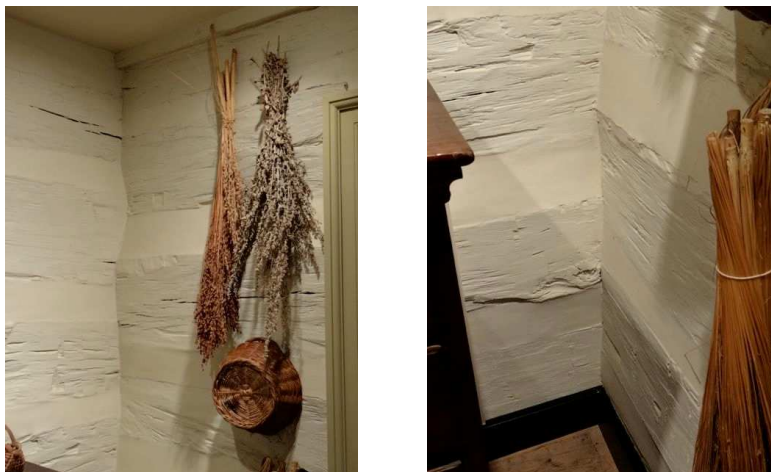
Original hewn logs, left visible here.
