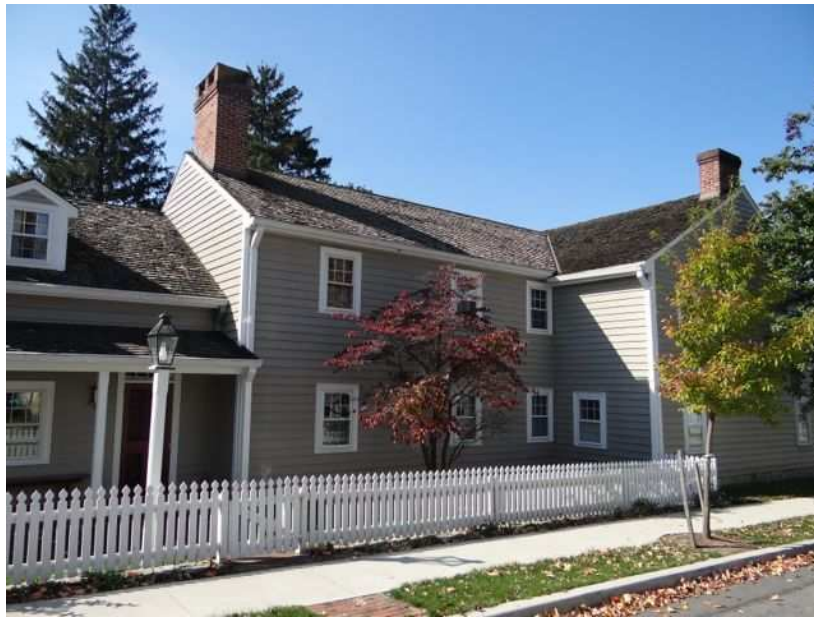
View from the side. The center and left-hand structures are later additions to the original structure.
