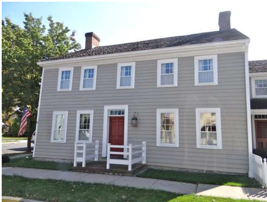
Front façade, showing the asymmetry of the window placement
