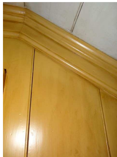
Wall boards beaded at the edges
