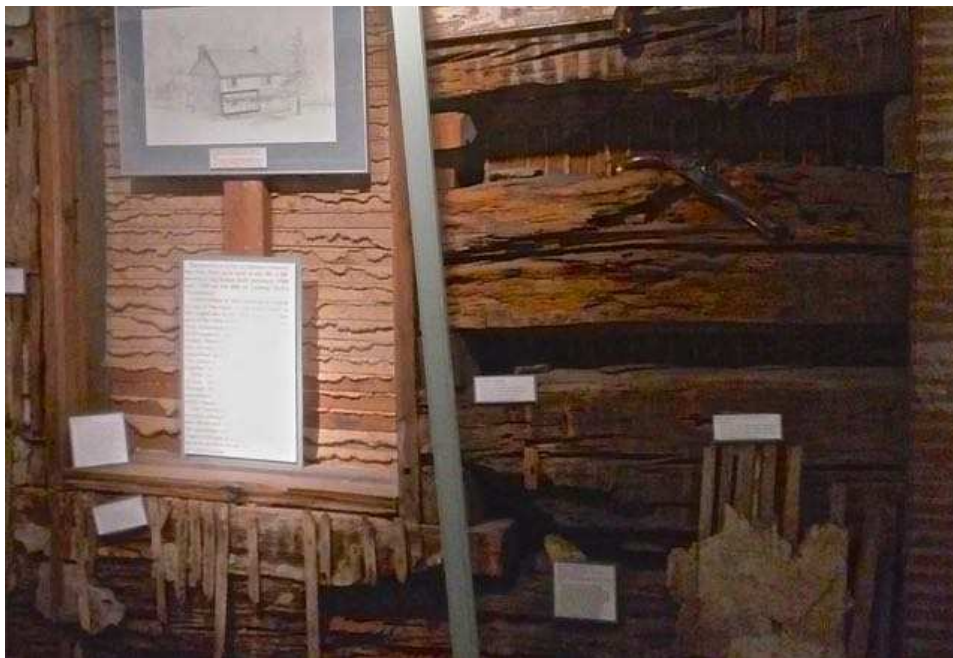
This log wall was discovered while some repairs were being done in the Packwood House Museum in the 1980s. The logs are part of the original log tavern built at the corner of Market and Water streets by about 1800.
