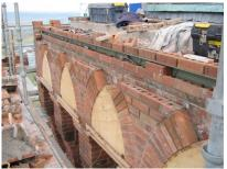
cotta accents. After nearly 75 years in service, the tower required much needed masonry repairs to extend its service life. The Bureau of Prisons had the foresight to preserve this asset due to its landmark status in the community, as opposed to full-scale demolition and/or truncation.
